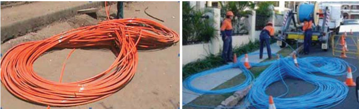
**Figure 7 Cable stored in 'fig-8' shape**
